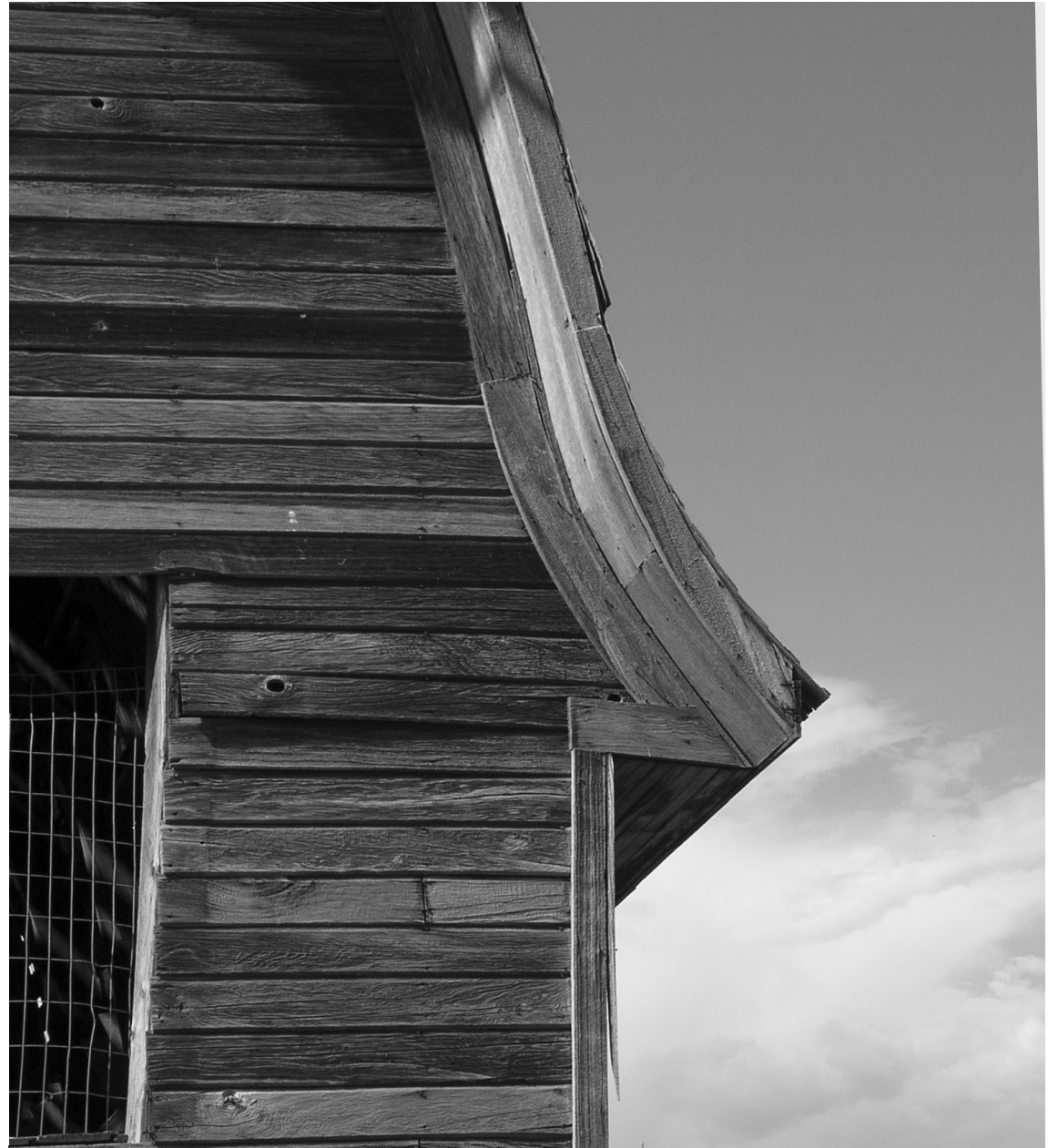
Left: Photo by Angela I. Nielson. Above: The gracefully curved bottom edge of the roof may have been practical in directing water away from the foundation, or it may have been simply decorative.
