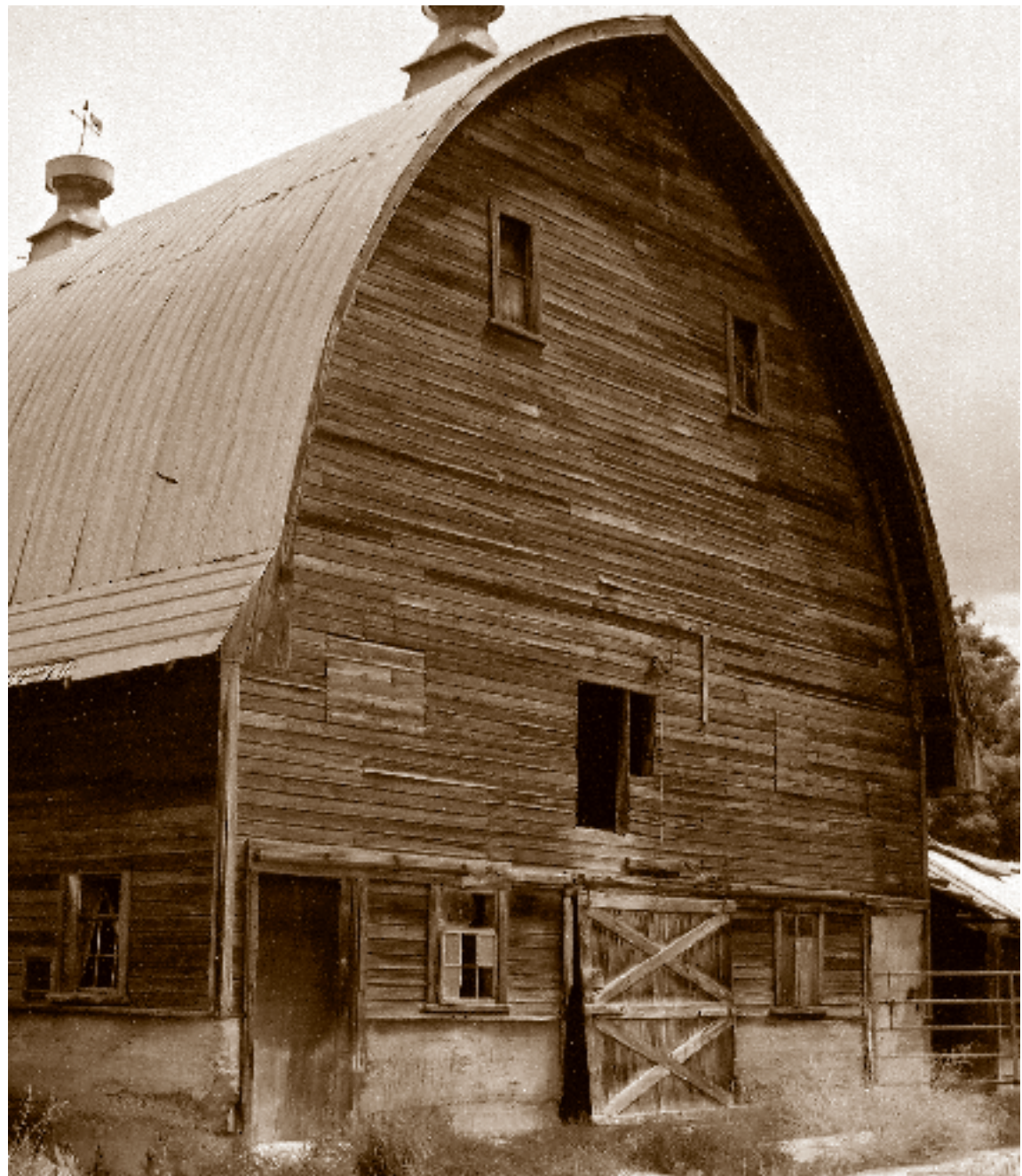
A large dairy barn in Richmond.
